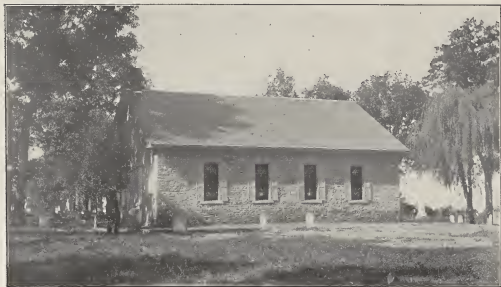
WYANDOT MISSION CHURCH RESTORED, 1889
